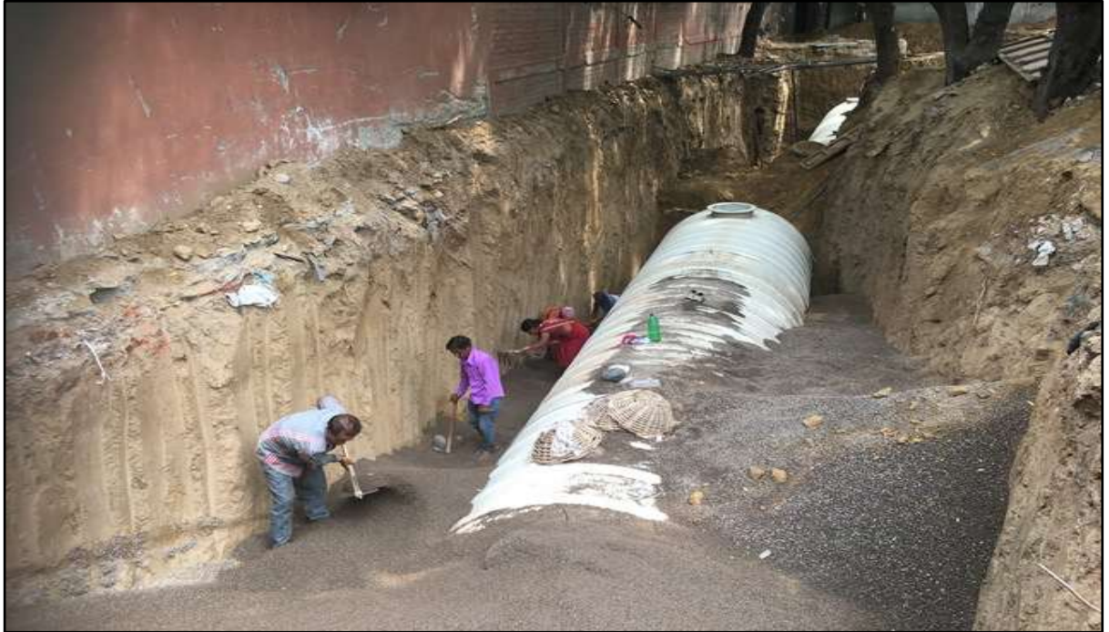
Gravel Filling of Sewer Treatment Plant
