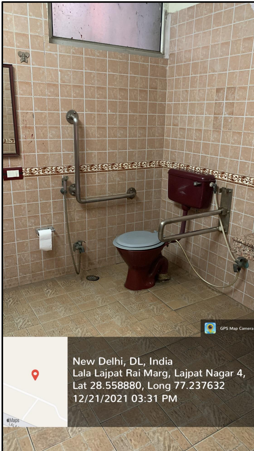
Washroom for Persons with Disability
